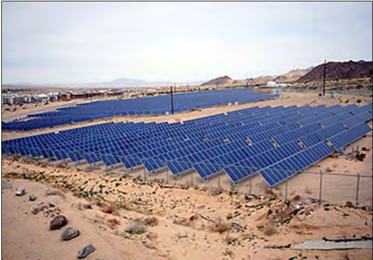
Photo 3. Existing Solar PV System at the Combat Center, Twentynine Palms
