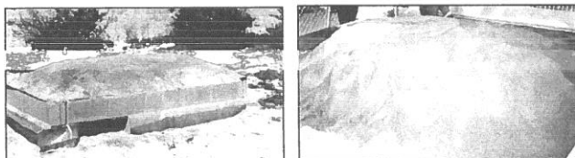
Figure 19. Aboveground burrow. (Left) Front view of completed structure shows opening. (Right) Rear view shows one foot of soil covering structure for adequate insulation.
