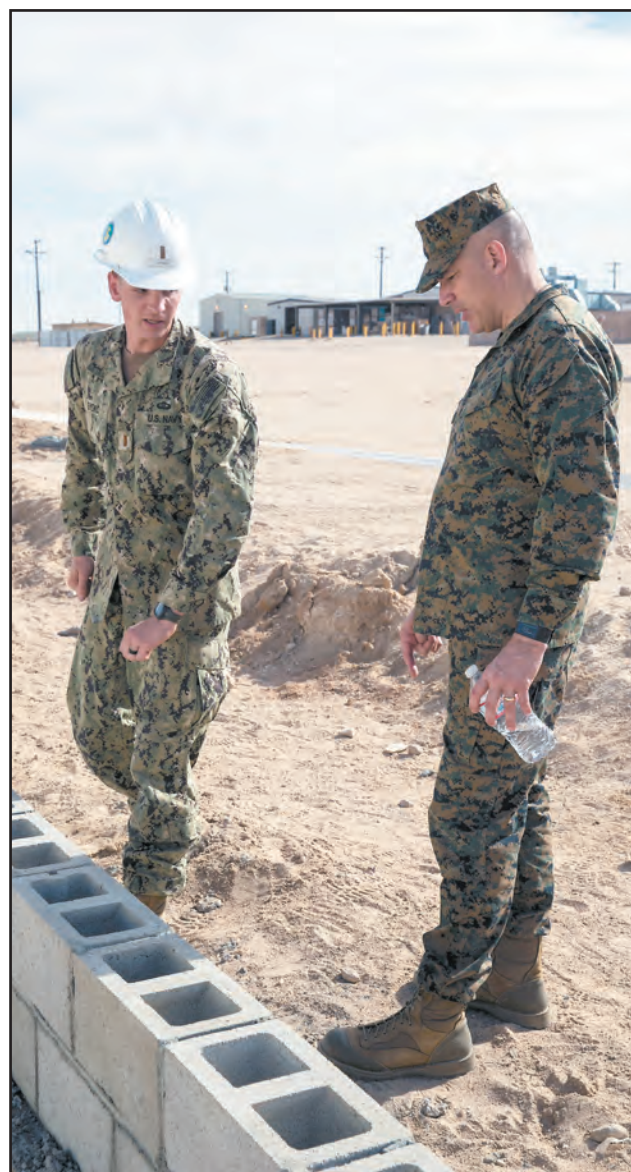
Ensign Frank Sysko, detachment Twentynine Palms Officer in Charge, Naval Mobile Construction Battalion 3, and Brig. Gen. William F. Mullen III, Combat Center Commanding General, tour the construction of the diversion walls in progress at Camp Wilson aboard Marine Corps Air Ground Combat Center, Twentynine Palms, Calif., Feb. 2. NMCB 3 is in Camp Wilson for three weeks working on the construction of displacement walls and K-Span units for their upcoming deployment in April.
