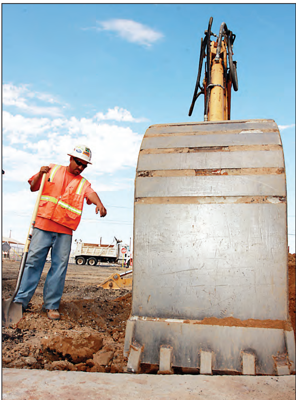
Adrian Navarro, a general laborer with Reyes Construction, points out areas of concern to Glenn Redmond as he operates a backhoe, Aug. 3, while working on a new parking lot at the Combat Center. The Helmets to Hardhats program is designed to help transitioning service members find careers in the construction industry.
