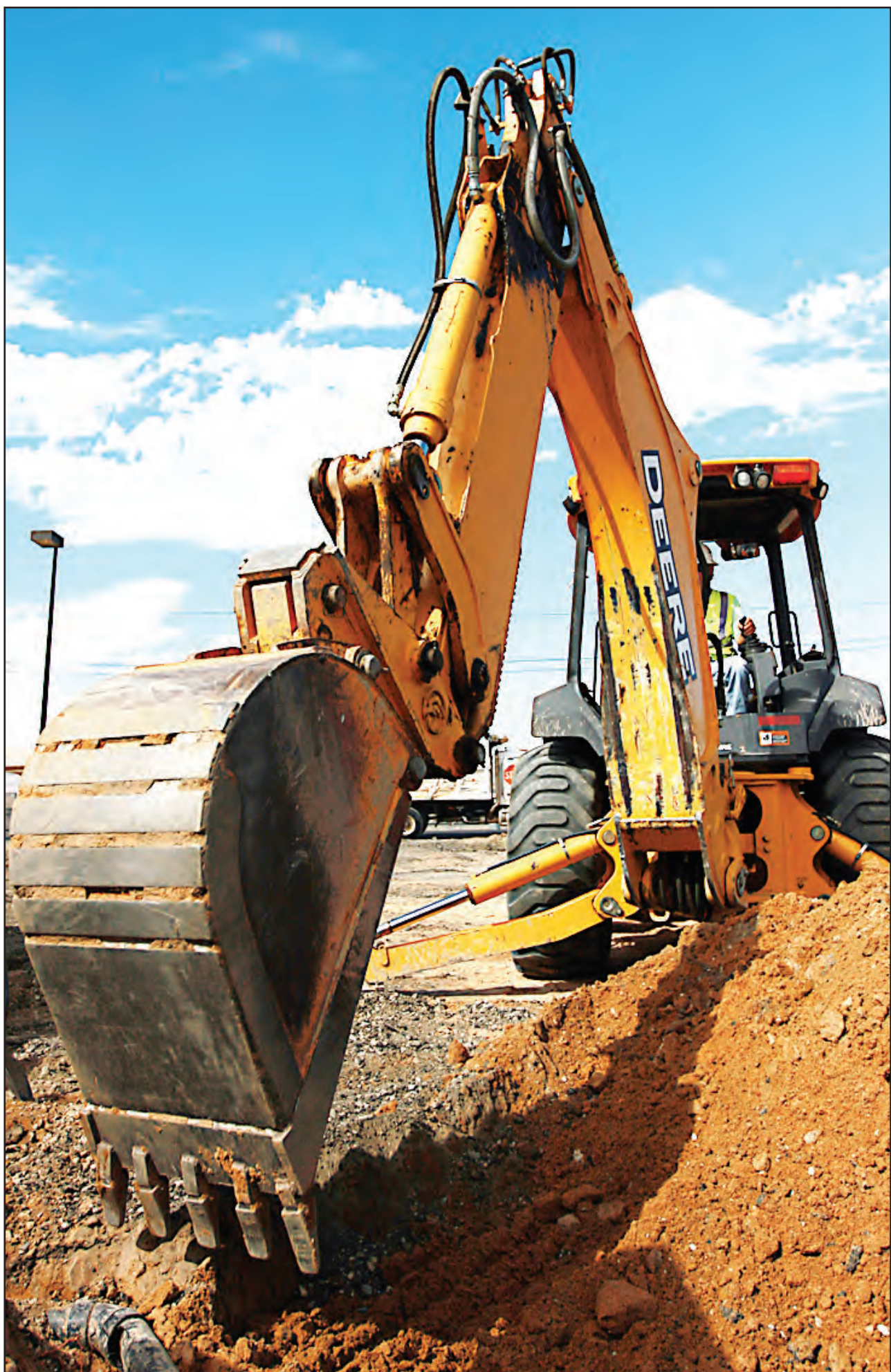
Glenn Redmond, a backhoe operator for Reyes Construction, smooths out ground to build a new parking lot at the Combat Center, Aug. 3. The Helmets to Hardhats program is designed to help transitioning service members find careers in the construction industry.
