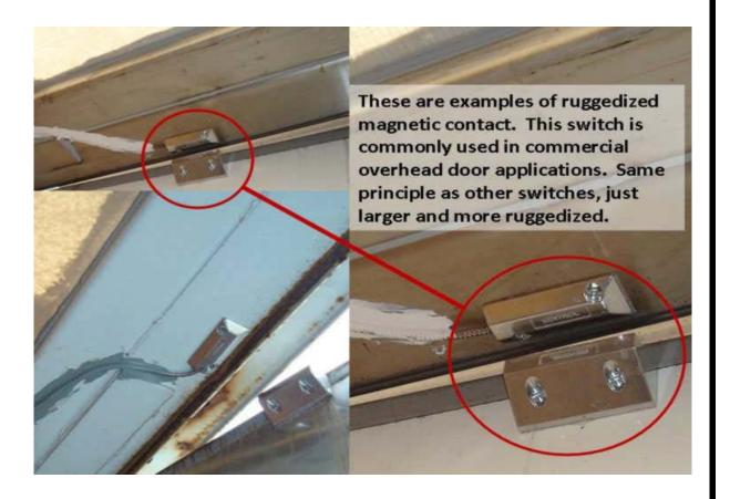
FIGURE 8-7. Trailer Tracking Door Contacts (Industrial)
