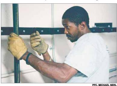
Monteray Bohannon, a rigger/installation technician with San Diego Stage and Light and a native of Kansas City, Mo., works to install new tracks for the support wires going into the Combat Center's Sunset Cinema Wednesday.
