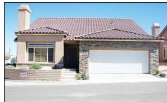
Plan 3B 3 bedroom, 3 bath, (Loft guest suite) 1840 Sq. Ft., Two-Car Garage, Family Room. Starting at $253,990
