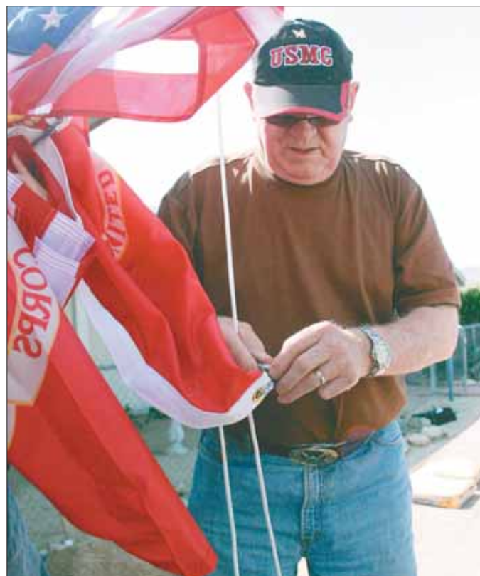
CPL. NICOLE A. LAVINE Korean War veteran Richard N. Blasongame attaches the Marine Corps flag to his new flagpole that was constructed by three Marines of 3rd Combat Engineer Battalion, Wednesday.
