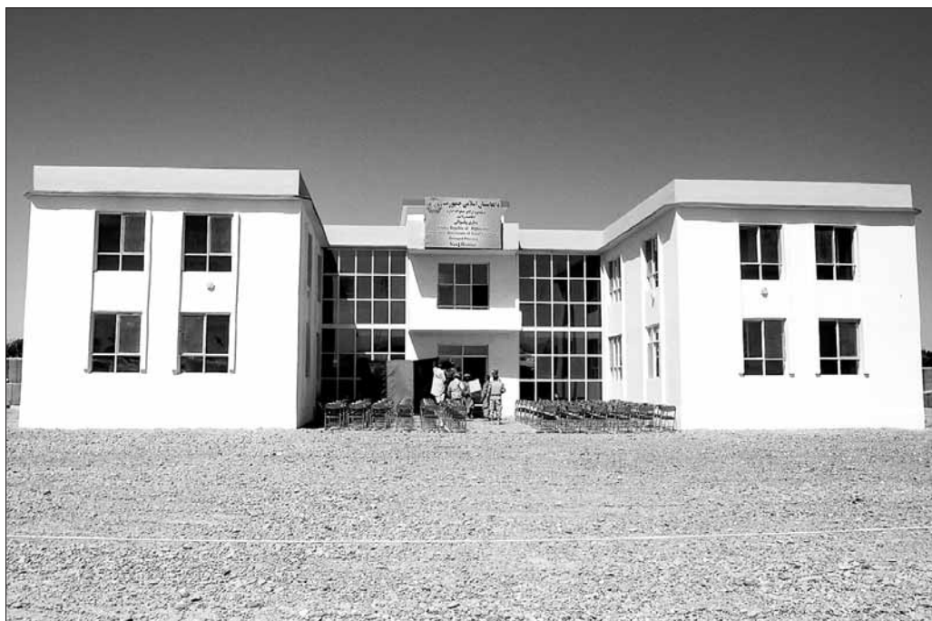
Pictured is a front view of Nawa, Afghanistan's new District Governance Center, hours before the building was officially opened in a ceremony April 18 by Helmand Provincial Governor Gulab Mangal and local government leaders from Nawa.
