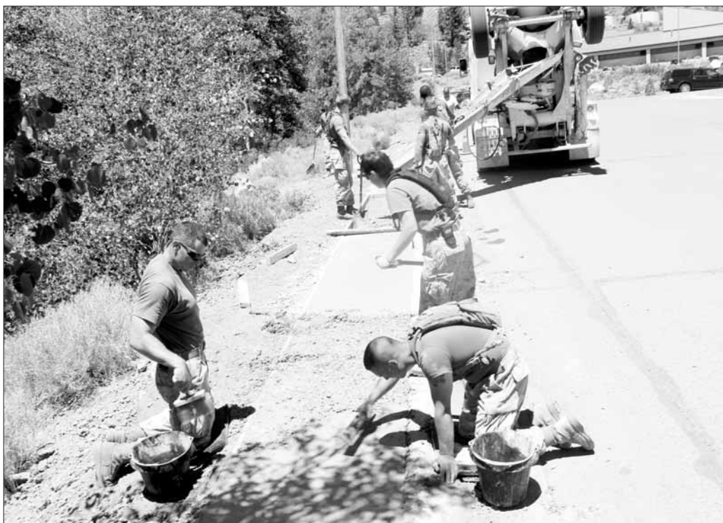
Marine engineers smooth out the still-damp concrete for a new sidewalk.
