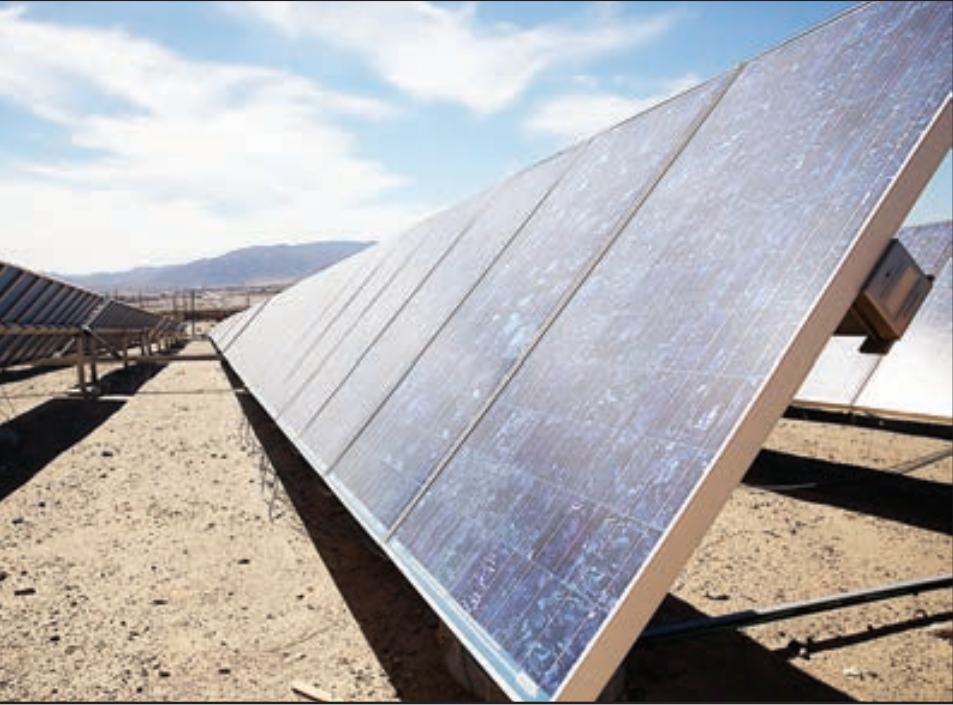
Several 1.2 megawatt, photovoltaic arrays are located in several areas aboard the Combat Center. These solar panels collect energy which is stored in a battery storage system.
