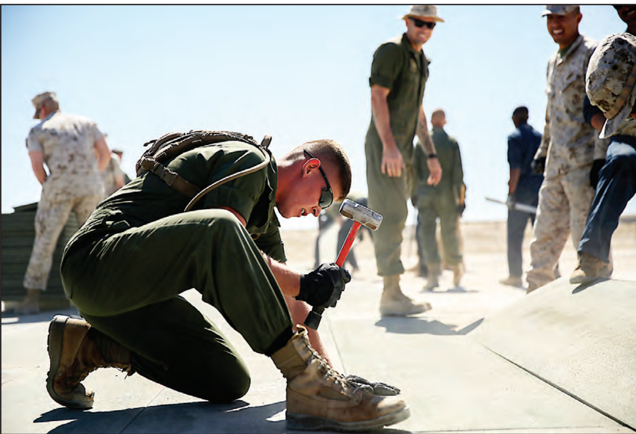
Lance Cpl. Tanner J. Clayson, Expeditionary Airfield Systems Technician, Marine Wing Support Squadron 372, pounds an aluminum panel into place during a refurbishing project on the Strategic Expeditionary Landing Field at Camp Wilson, Monday.
