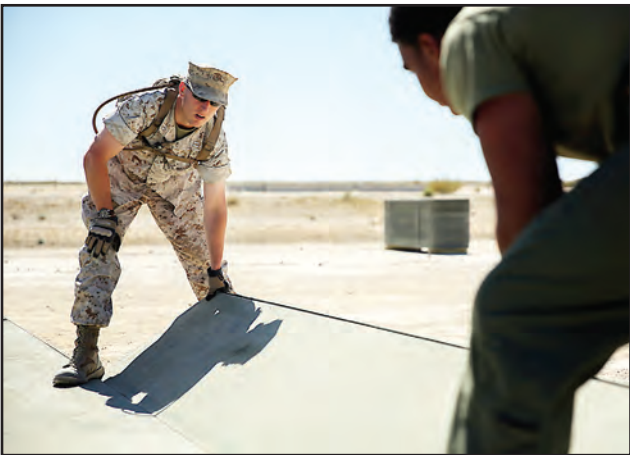
Capt. Christian Carlson, Motor Transportation Company Commander, Marine Wing Support Squadron 374, assists a Marine with an aluminum panel that is a part of the new matting on the Strategic Expeditionary Landing Field at Camp Wilson, Monday.
