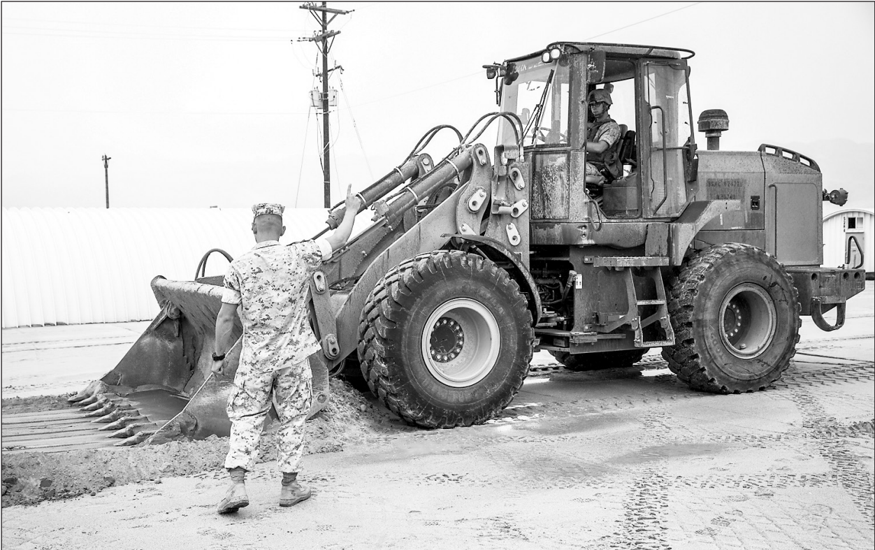
Marines with Combat Logistics Battalion 7 lay the foundation for additional expeditionary steel structures, known as K-Spans, at Camp Wilson aboard the Combat Center, Sept. 23.
