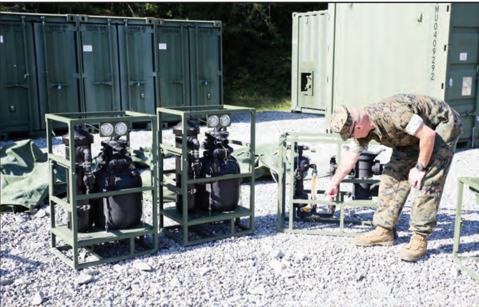
Master Sgt. Ryan Miller, project officer for Family of Water Systems at Marine Corps Systems Command, assembles the Lightweight Water Purification System with the new Enhanced Production Module.
